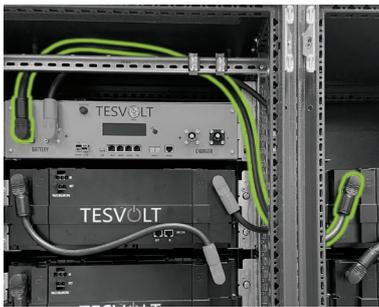
Connect the last module and the APU HV1000-S using the connecting cable (3.2). Make sure you follow the instructions in section "5.7 Wiring the battery modules" on page 20.
