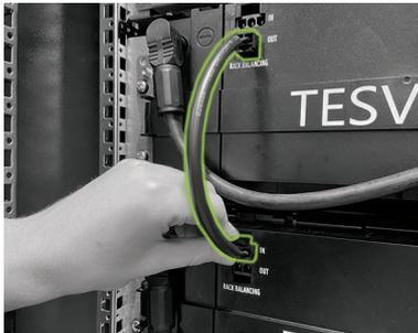
Connect the rack balancing "OUT" connection (2.2) of the first battery module below the APU HV1000-S to the rack balancing "IN" connection (2.1) of the next battery module down using a rack balancing module connector (4.3). Continue in this manner, connecting all the battery modules in the left half of the cabinet.
