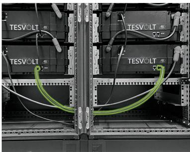
Establish the BAT-COM connection between the bottom battery modules using the longer patch cable (5.2).
