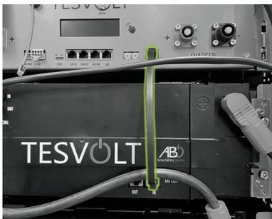
Connect the BAT-COM communication cable using the the supplied patch cables (3.3), (4.2) and (5.2). Connect the "BAT-COM" (11) connection of the APU HV1000-S and the BAT-COM "IN" connection on the battery module positioned below the APU HV1000-S using a patch cable (3.3). Then use a patch cable (4.2) to connect the same module's BAT COM "OUT" connection to the next module's BAT-COM "IN" connection.
