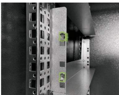
Now, fit the cage nuts (J) for fastening the battery modules (2) with the auxiliary tool (J1) (see "5.7 Wiring the battery modules" on page 20 et seq. for the positions of the battery modules). Distribute the cage nuts from bottom to top. Start at the bottom edge of the slide rail for the relevant battery module. Fit the first two cage nuts in the second opening on both sides from below, and fit the remaining two cage nuts in the top opening in the two slide rails.
