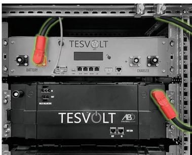
The battery modules of the TS HV 70 are connected in series. The colours of the plugs must match the colours of the jacks on the battery module, i.e. red plug to red jack, for example. Start on the left side of the cabinet with the APU HV1000-S and the first battery module and the connecting cable (3.1).
