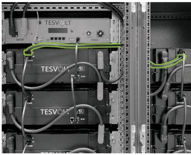
Now connect the remaining battery modules on the right side, starting from the bottom. Follow the specifications in section "5.7 Wiring the battery modules" on page 20 et seq.
