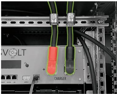
Only connect the DC cables (7.1) and (7.2) to the HV1000-S APU once the SMA STPS 60 is completely connected.
