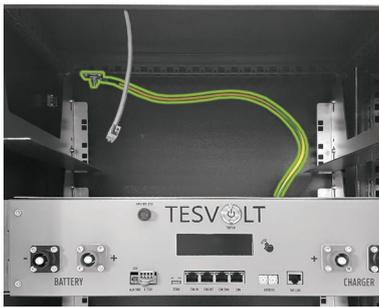
Attach the end to the central grounding point (C) with the M8 ring cable lug. Use a torque wrench with a tightening torque of 10 Nm. For easier installation, you can temporarily place the APU HV1000-S on the slide rails of the first battery module during installation.
