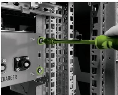
Insert the APU HV1000-S in the left half of the cabinet on the top-most slide rails and use the enclosed M6 x 16 pan head screws (I) (cross-head) and plastic washers (I.I) to fasten it to the pre-installed cage nuts (J).
