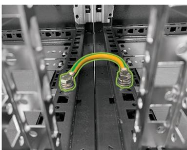
Fit the prepared grounding cable (M.6) to the middle cabinet frame profiles using the pre-fitted speed nuts (M.5). Use a torque wrench with a tightening torque of 10 Nm.
