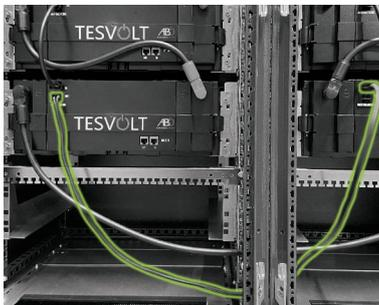
Use one of the 1.10 m long rack balancing connecting cables (5.3) to connect the bottom modules in the left and right halves of the cabinet.
