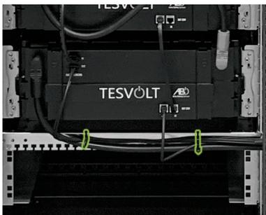
Fasten the cabinet connector cables in the bottom part of the cabinet to the cable retention rails (F) using cable ties.
